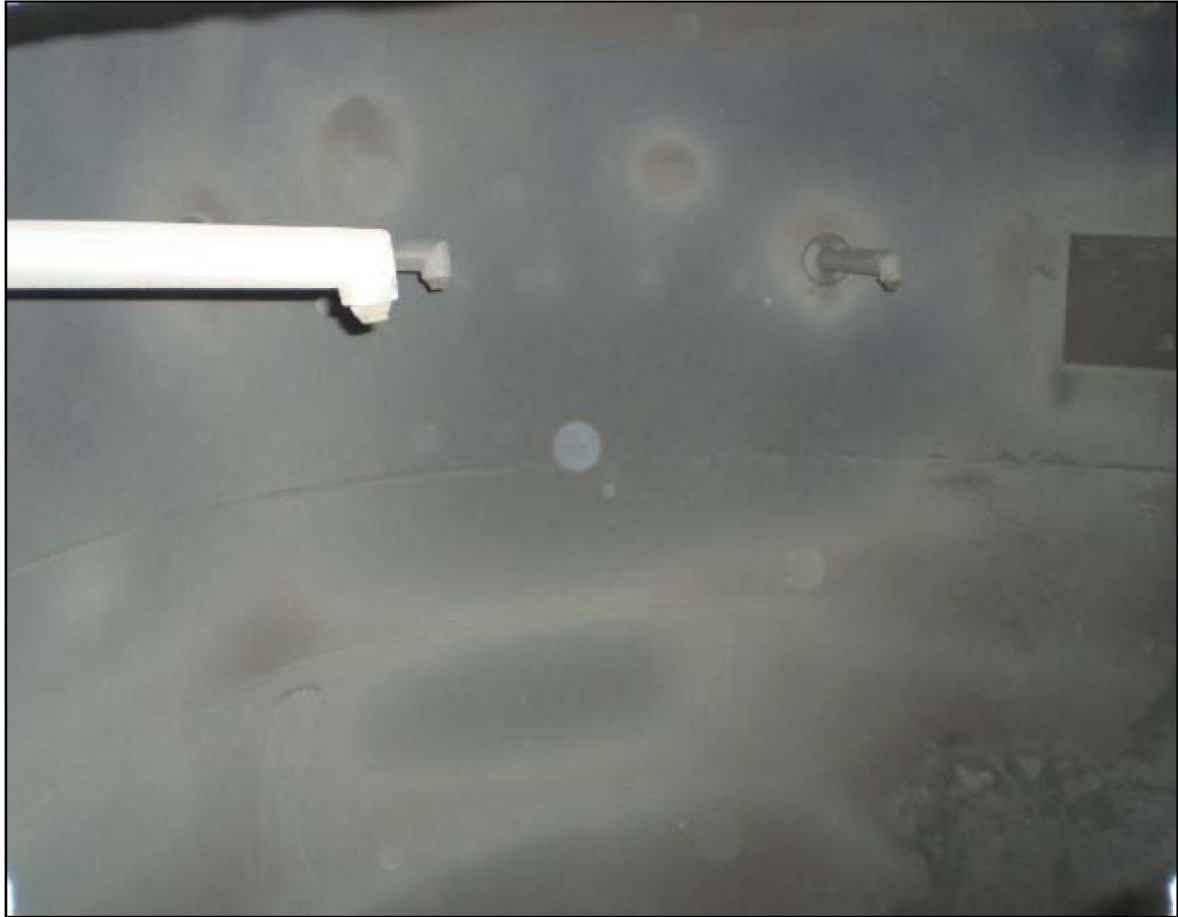
Pic. 9: Spray nozzles inside of spray absorber
