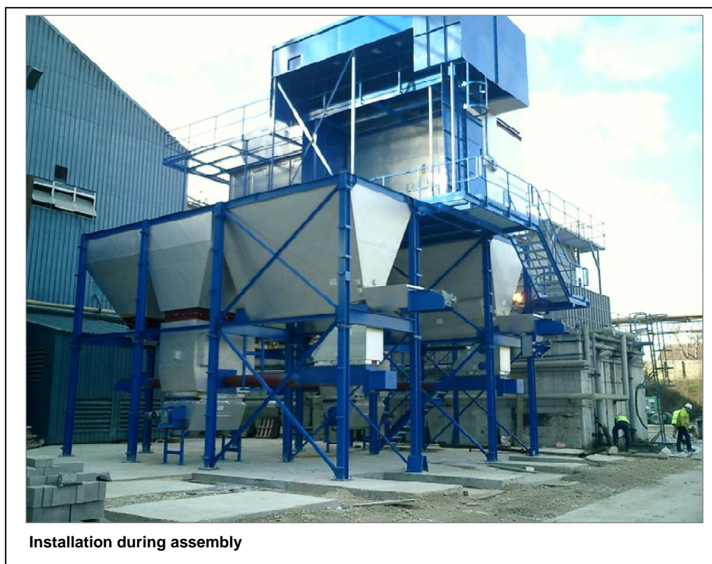
Pic 13: Application example Fabric filter downstream tank for container glass
