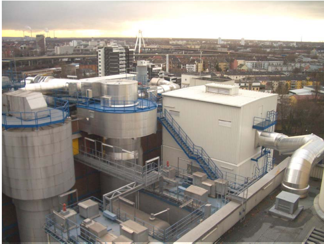
Illustration 2: MHKW Ludwigshafen crude gas cleaning line 2 Spray absorber head and filter / reactor building
