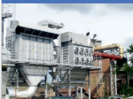
Flat-tube heat exchanger without cooling air recirculation
