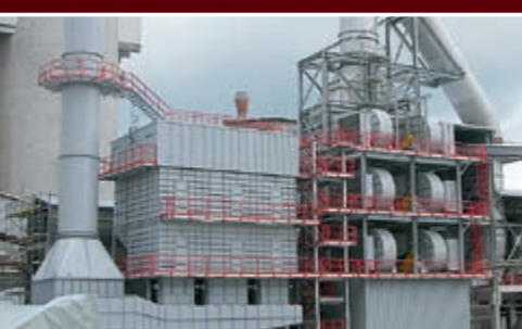
Flat-tube heat exchanger
